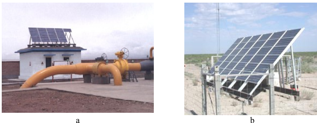
Picture 1. Objects of main transport of gas (a) and oil (b) with photo-electric systems of power supplies of cathodic protection stations
